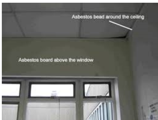
Asbestos panelling
