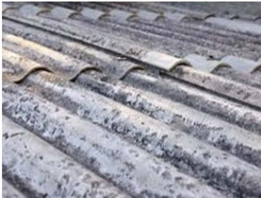
Asbestos cement roof
